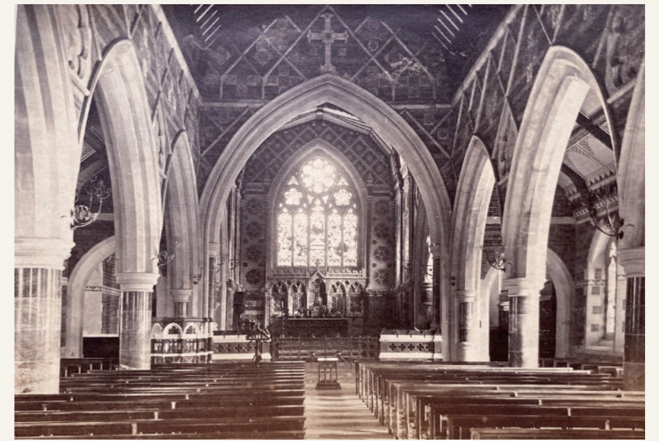
Fig.3 Cabinet half-plate albumen print, undated, unsigned and untitled, showing the church as it was not long after completion in 1873. Collection of the author.
